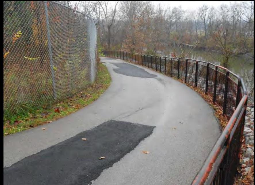
This project will address river bank failure located between the Tennessee River and the Will Skelton Greenway asphalt-paved walking trail, below the Tennessee School for the Deaf. The failure extends into the paved greenway trail and must be stabilized as soon as possible.
