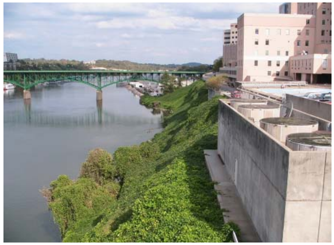
LOWER SECTION - Area 3-5 Looking east from Henley Bridge
