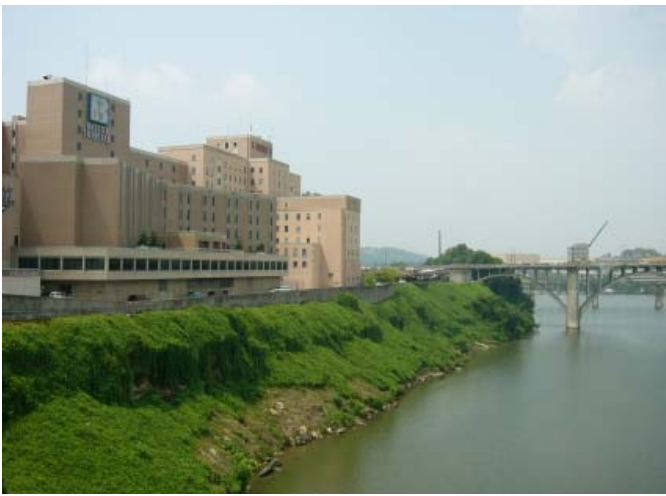
LOWER SECTION - Area 1-5 Looking west from Gay Street Bridge
