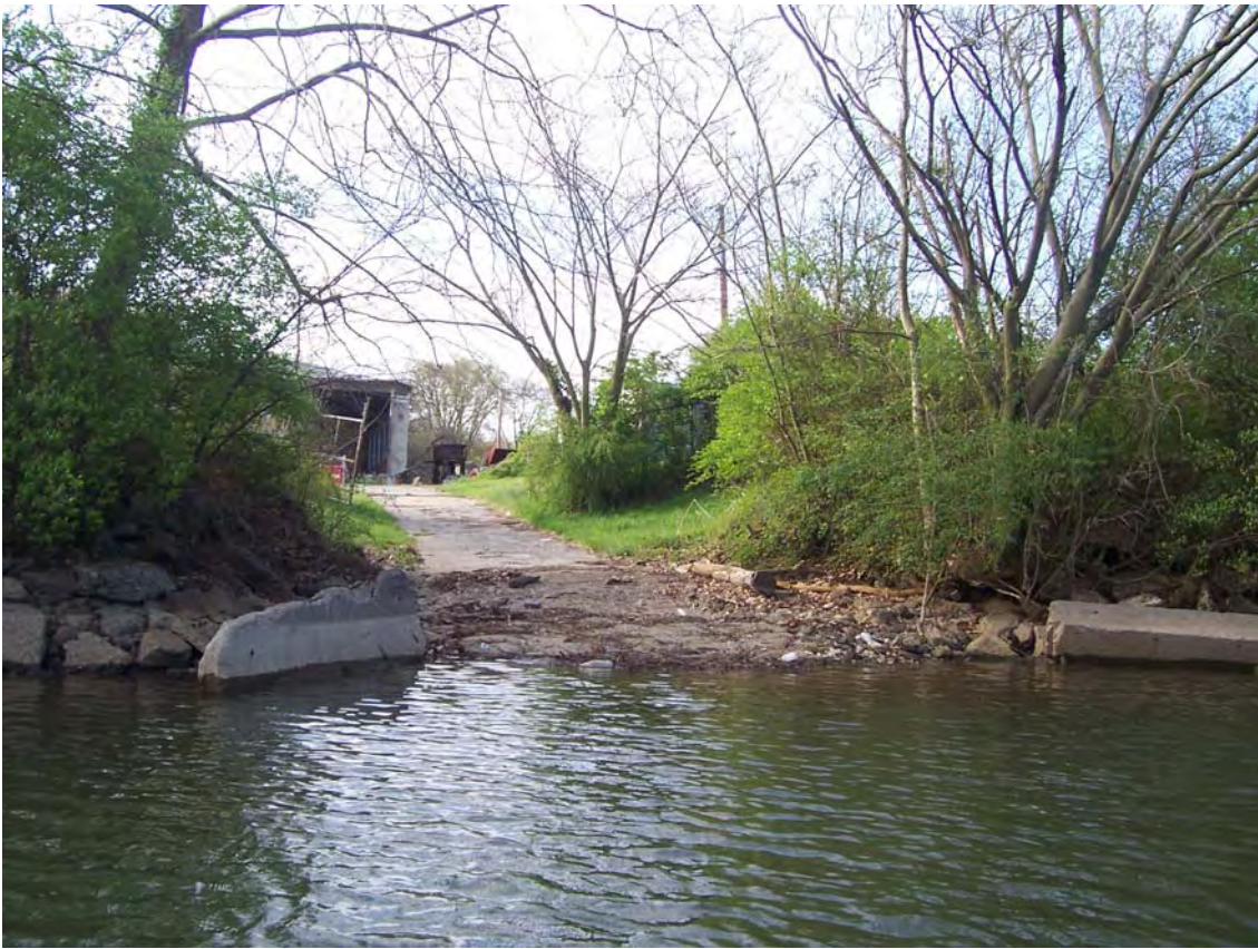
Photograph #BT-11. View to south. Boat ramp located on Project 10 site.
