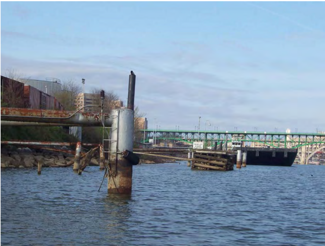
Photograph #BT-21. View to west of metal barge piers and wooden dock on Project 9 site.
