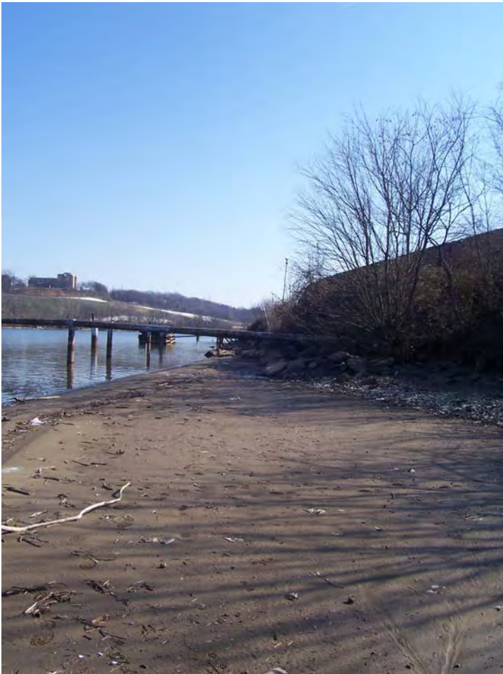
Photograph 9-56. View to east from shoal area towards metal piers.
