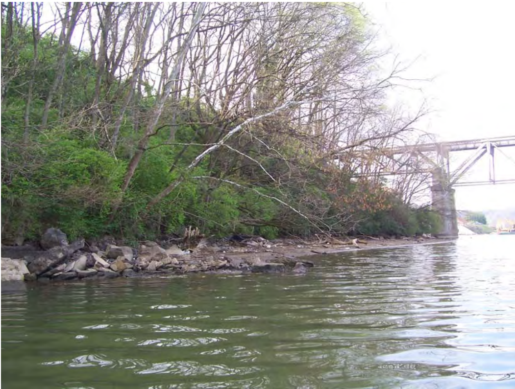
Photograph #BT-45. View to west of limestone bluff and shoals located between the Henley Street Bridge and Norfolk Southern Railroad Bridge in the Project 6 area.
