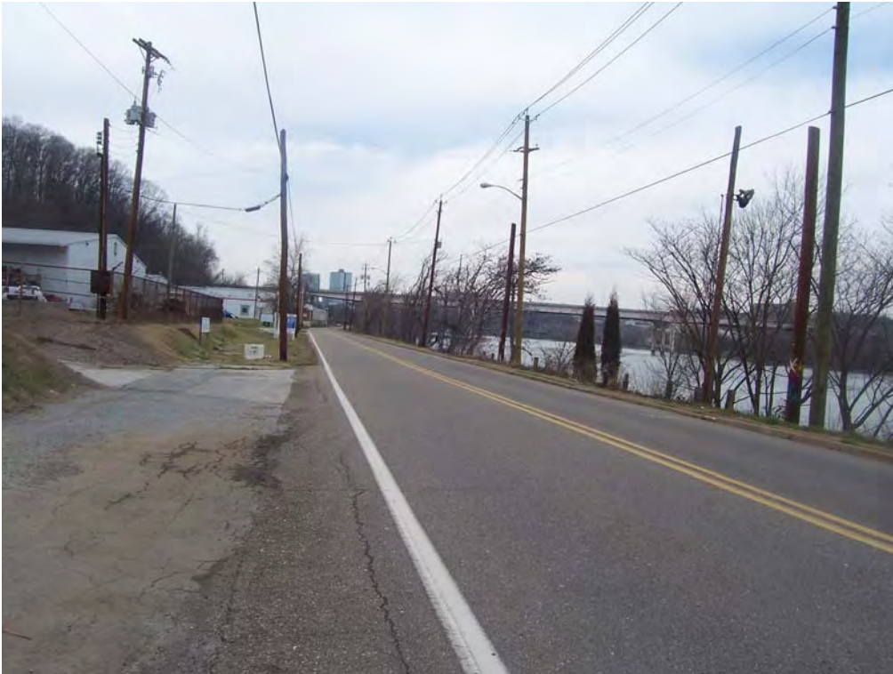
Photograph 11-1. View to northwest. Island Home Avenue towards South Knoxville Bridge.
