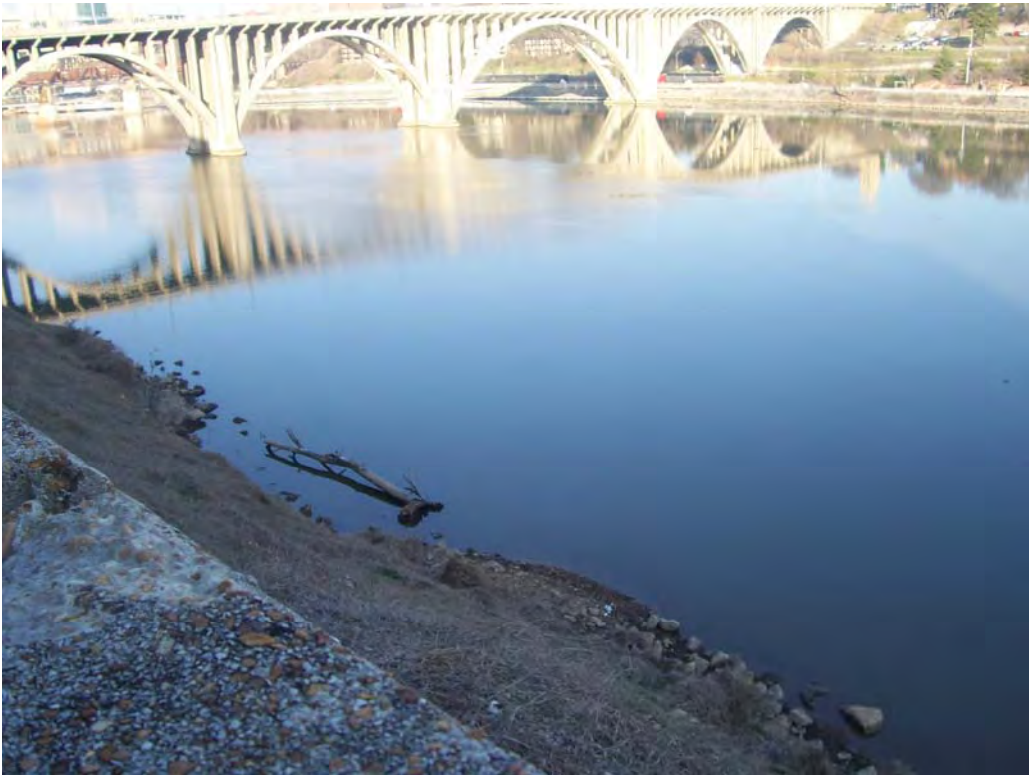
Photograph 6-8. View to northwest. Bluff and shoal area; Henley Street Bridge.
