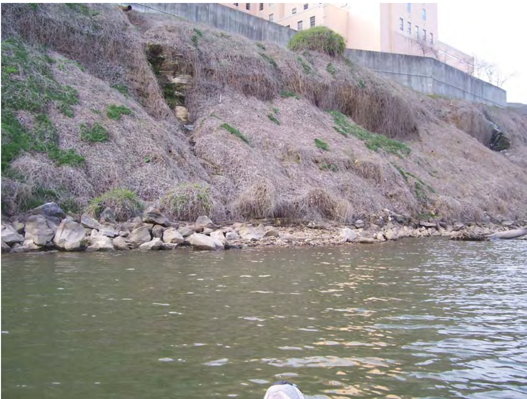
Photograph #BT-34. View to southwest of general stormwater drainage from Baptist Hospital onto bluffs. Continuous drainage has eroded limestone and permitted growth of mosses (just left of photograph's center). Shoal area evident in foreground.
