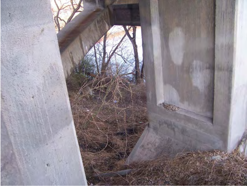
Photograph 6-17. View to northwest underneath Henley Street Bridge.
