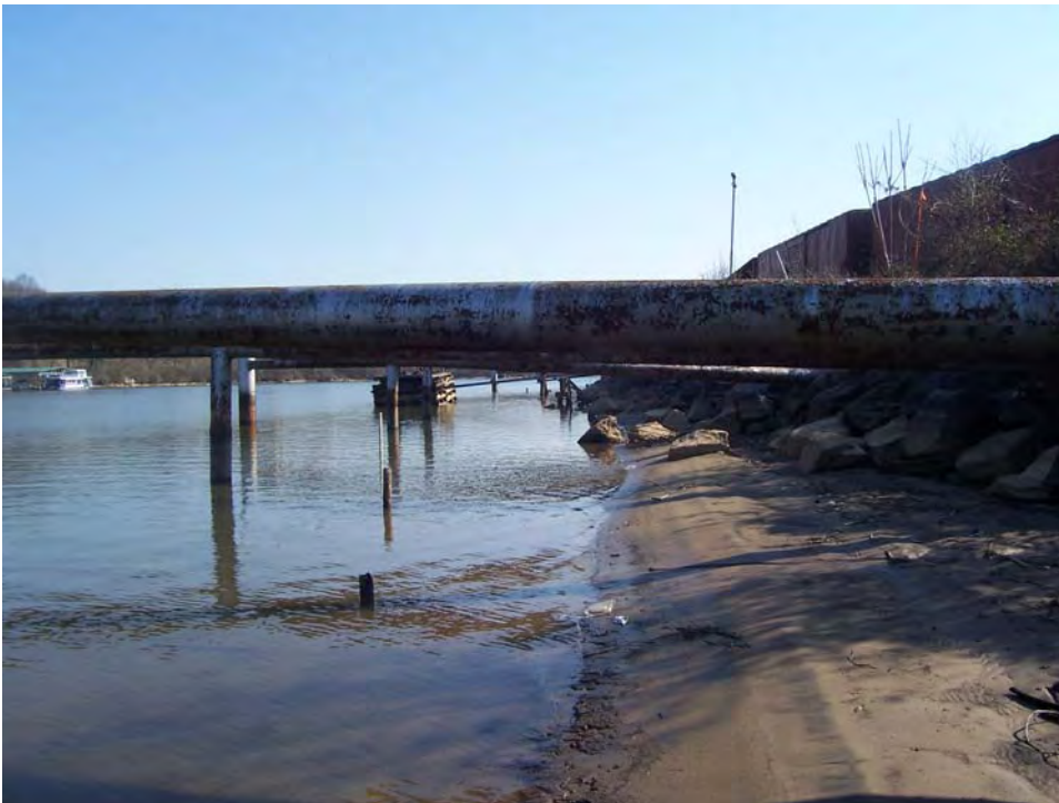
Photograph 9-58. View to east. Eastern end of shoal area near metal piers.
