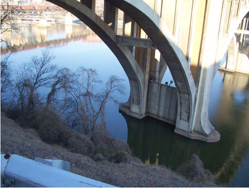
Photograph 6-15. View to northeast of bluff area and Henley Street bridge.
