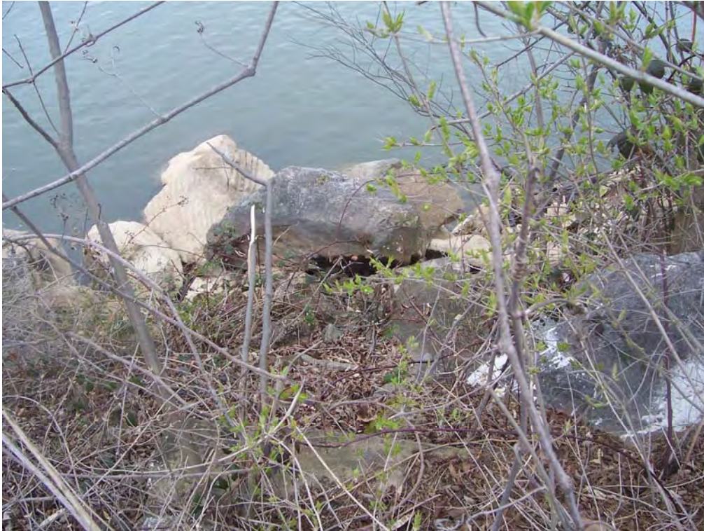
Photograph 11-7. View to north. Typical riprap and shoreline vegetation.
