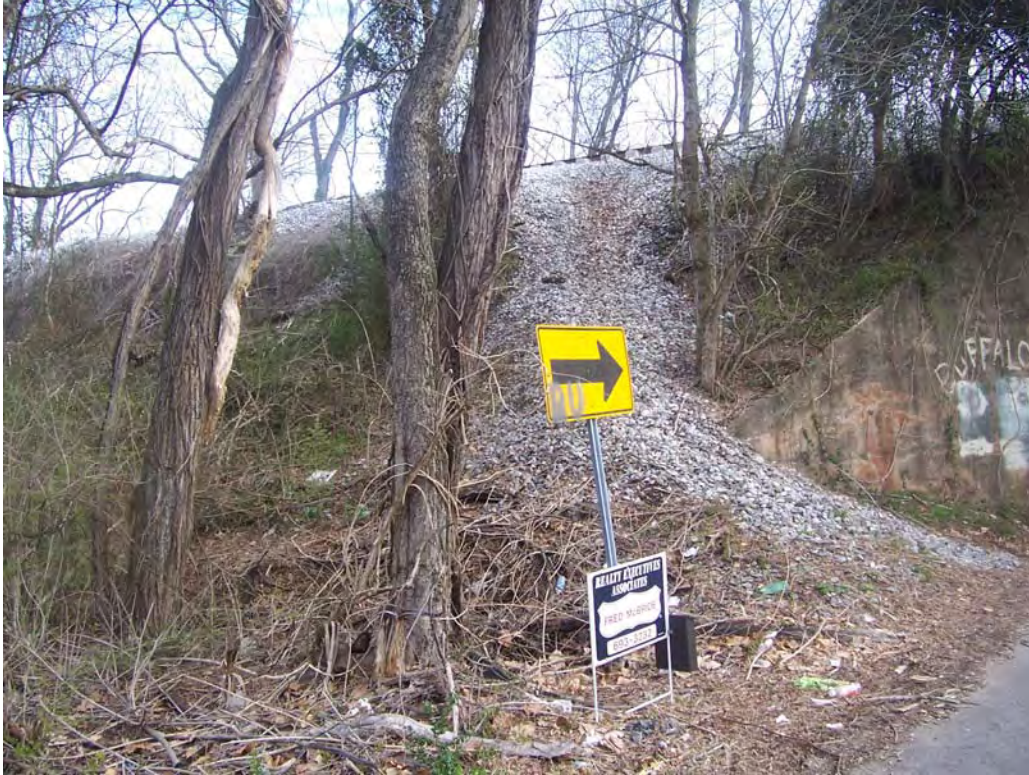
Photograph 1-1. View to east. West side of railroad underpass at Scottish Pike/Cherokee Trail intersection.
