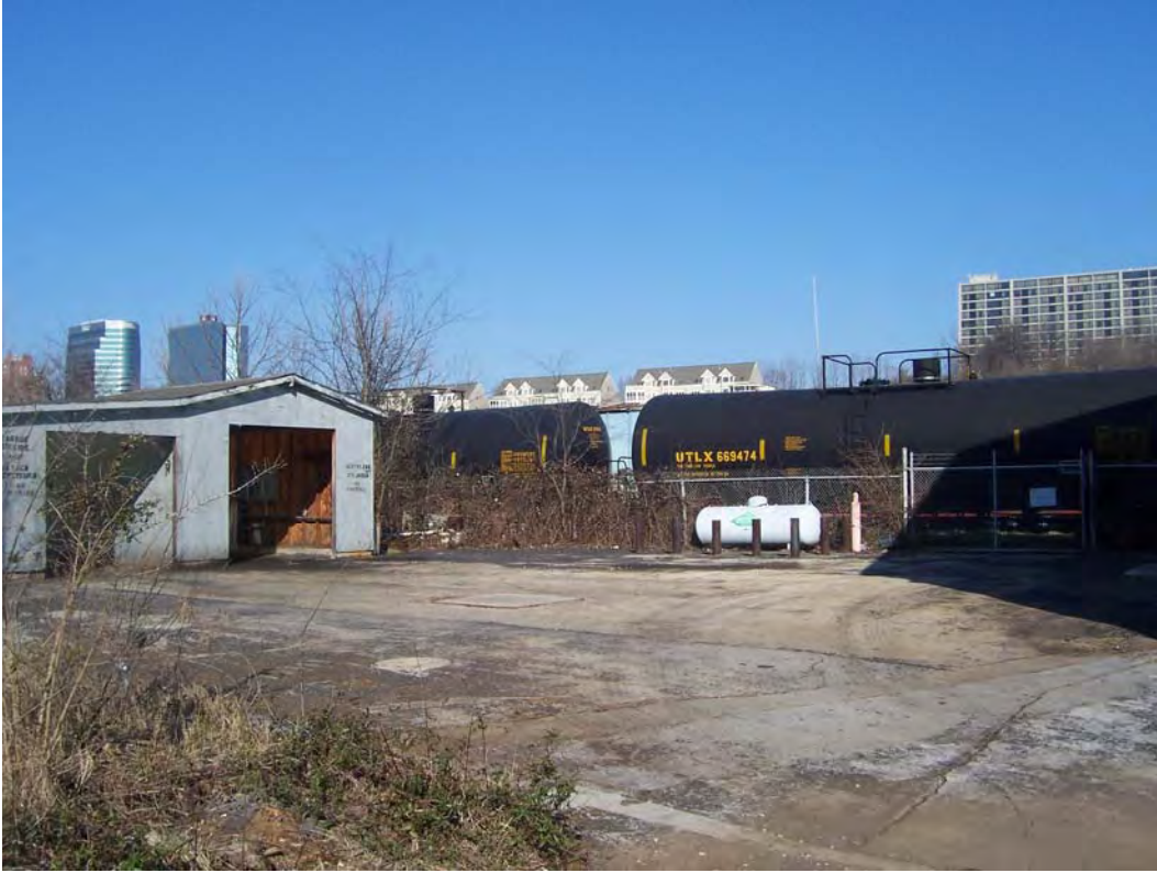
Photograph 9-7. View to northwest. Garage area west of main building.
