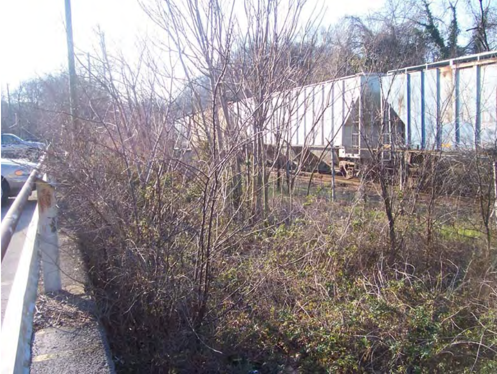
Photograph 5-3. View to southwest. Western border of parking lot adjacent to Norfolk Southern Railroad tracks.
