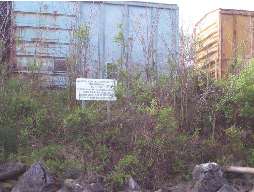
Photograph #BT-22. View to south of outfall for Industrial Stormwater NPDES permit TN0067156 for the former Star Enterprises fueling area on the Project 9 site.
