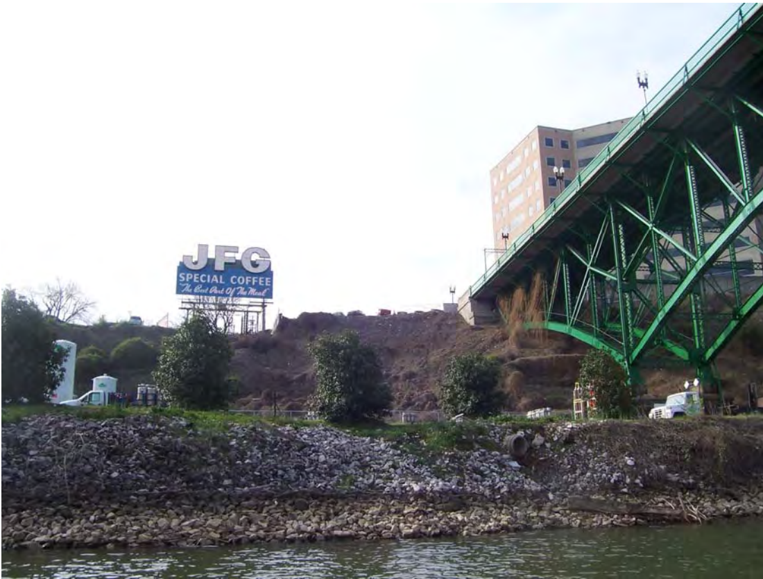
Photograph #BT-27. View to south of Project 7 area and Gay Street Bridge. Stormwater outfall from Holston Gas property.
