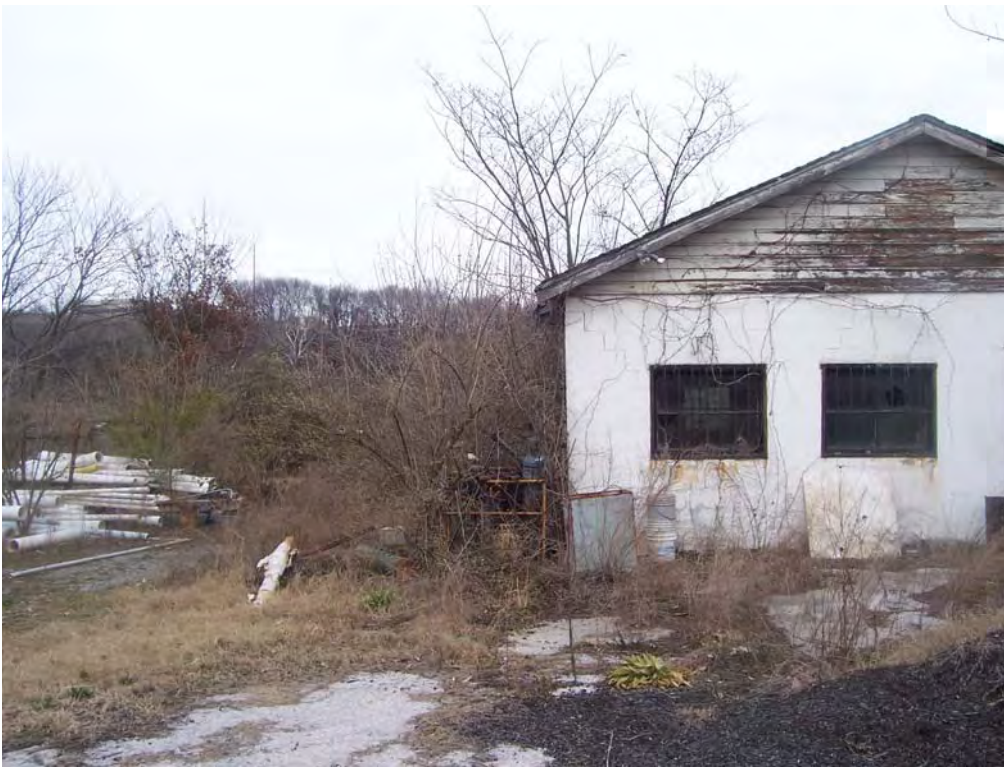
Photograph 10-21. View to west of storage building located south of metal barge pier. Note outside storage of equipment, drums, and gas cylinders.
