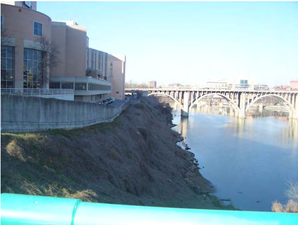
Photograph 6-2. View to west from Gay Street Bridge. Bluff and shoals area.
