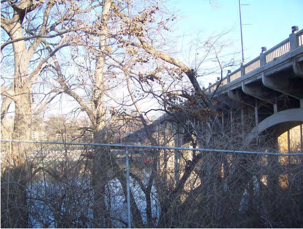
Photograph 6-19. View to northeast of Henley Street Bridge from parking lot.
