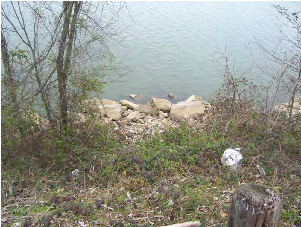
Photograph 11-8. View to north. Typical riprap and shoreline vegetation.
