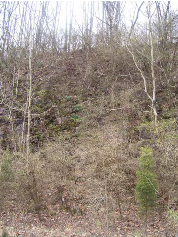
Photograph 12-22. View to west. Exposed limestone along western border of quarry area adjacent to railroad tracks and West Blount Avenue.
