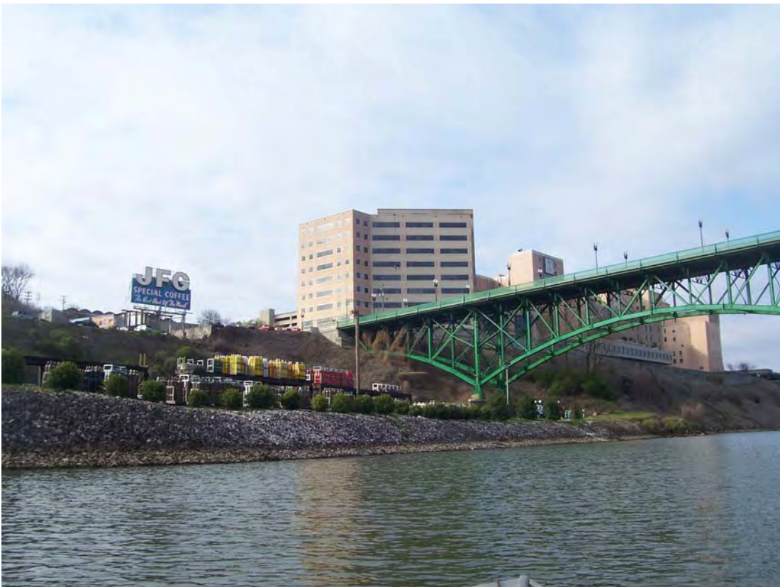
Photograph #BT-26. View to southwest of Gay Street Bridge and Project 7 area.
