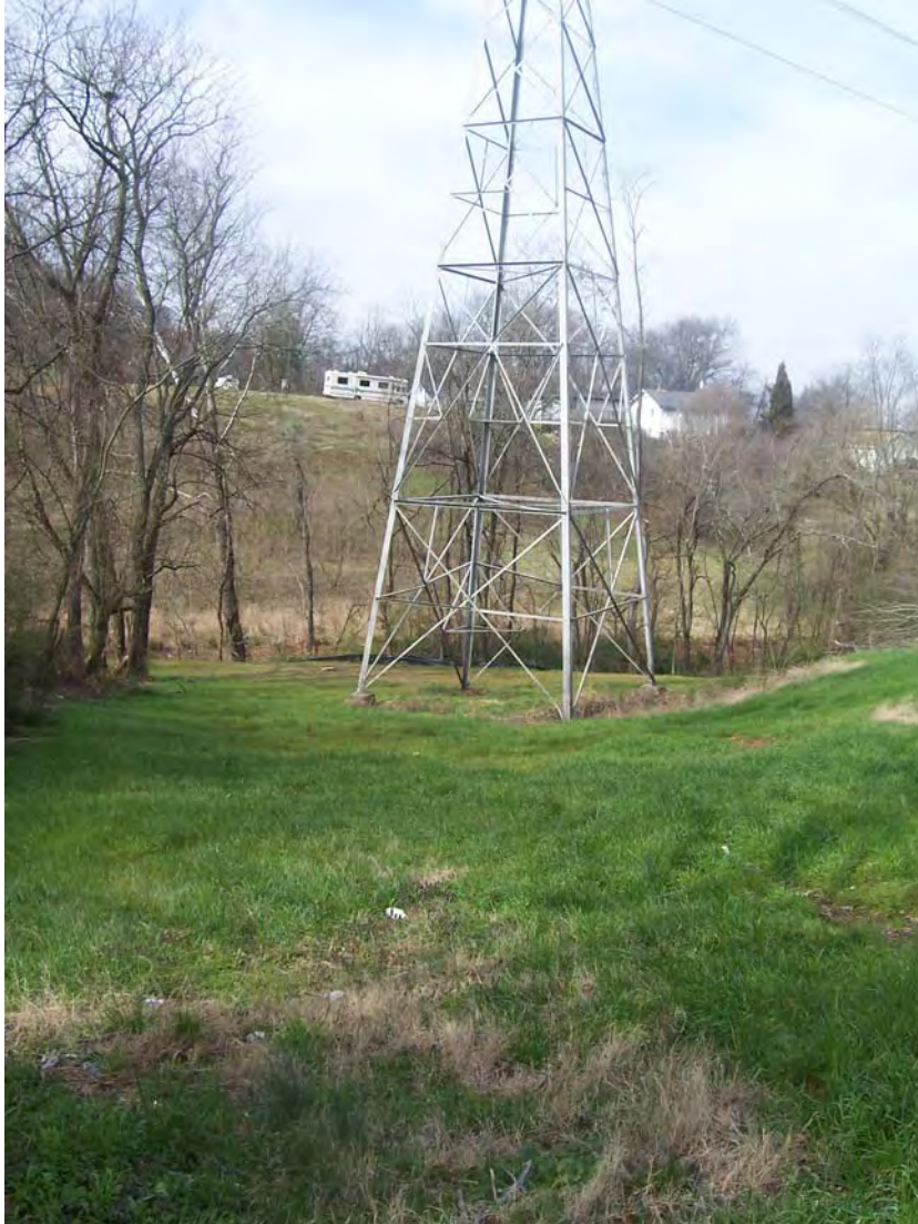
Photograph 1-31. View to west. City of Knoxville KUB property located between West Blount Avenue and the east bank of Goose Creek.
