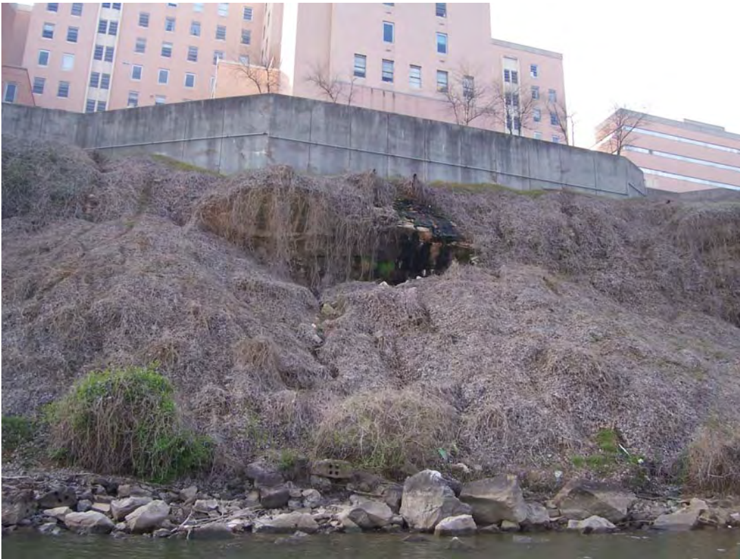
Photograph #BT-35. View to south. Project 6 bluff area and shoals. General stormwater drainage from Baptist Hospital onto limestone bluffs (area dark colored rocks) permits growth of mosses.
