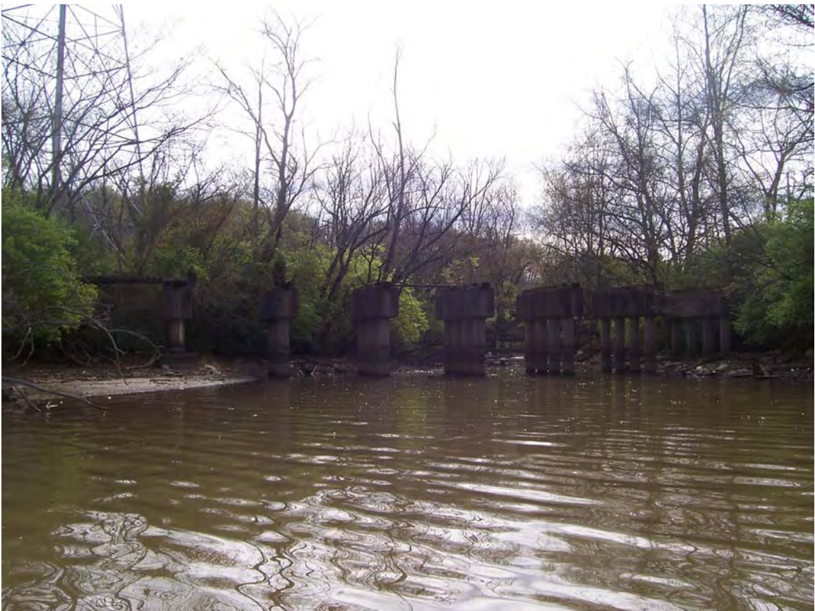
Photograph #BT-64. View to south of the mouth of Goose Creek.
