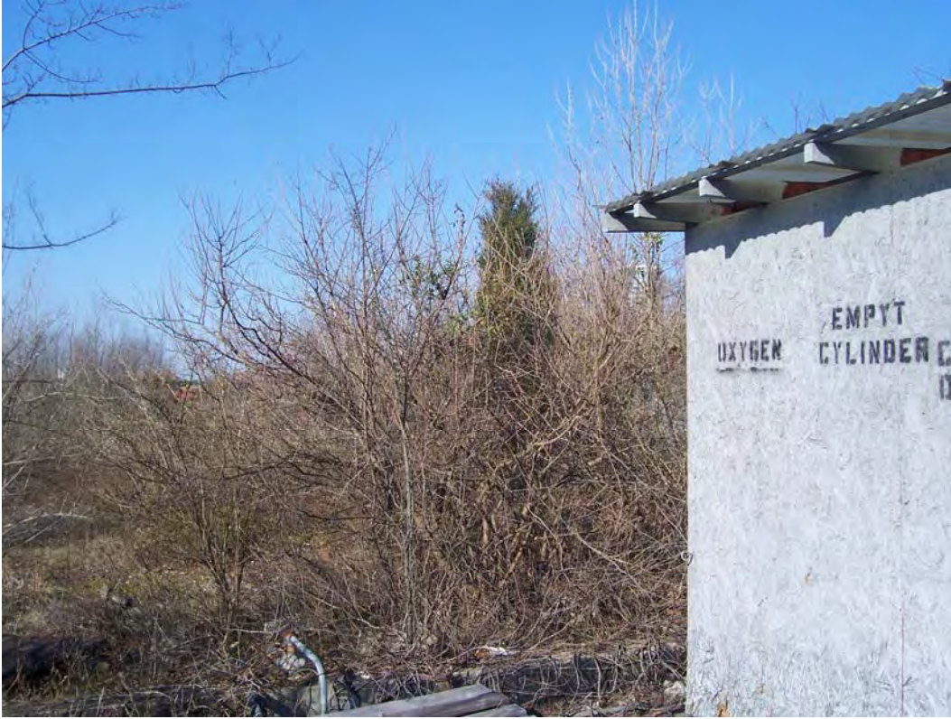
Photograph 9-11. View to northwest. Area adjacent to and behind garage.
