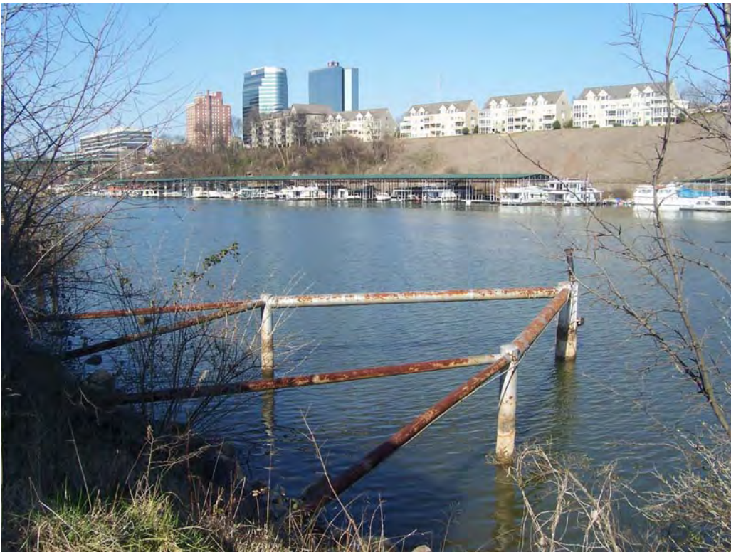
Photograph 9-44. View to northwest. Shoreline by eastern metal barge pier.
