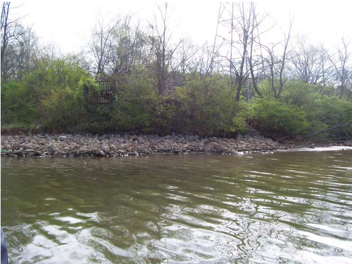
Photograph #BT-62. View to east of pipeline crossing and east bank of Goose Creek at its mouth.
