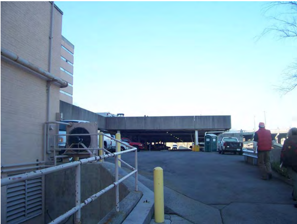
Photograph 6-10. View to west. Parking garage area between Baptist Hospital and Henley Street Bridge.
