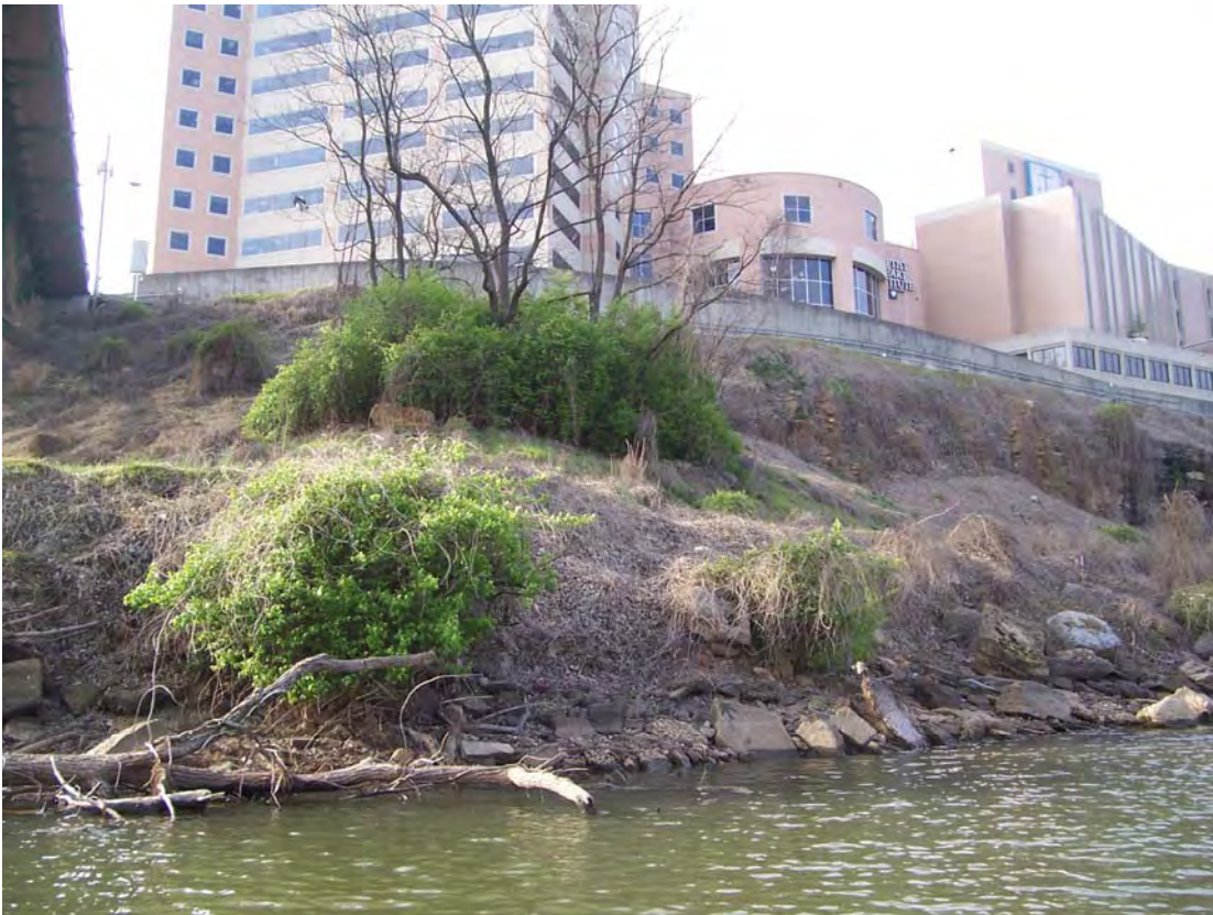
Photograph #BT-29. View to south of Project 6 area. Kudzu ( Pueraria montana ), an invasive species, covers the limestone bluff in front of Baptist Hospital. A large shoal area is located in this project area between the Gay Street and Henley Street Bridges.
