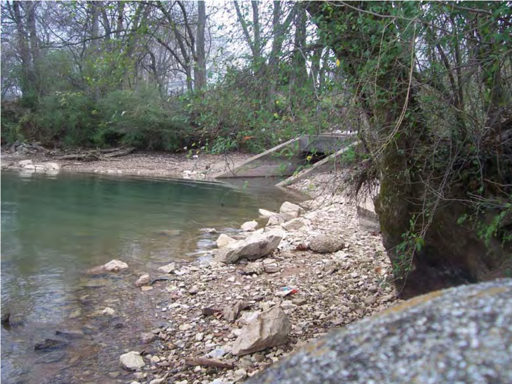
Photograph 11-14. View to southeast. Mouth of Baker Creek near entrance to Island Home Neighborhood.
