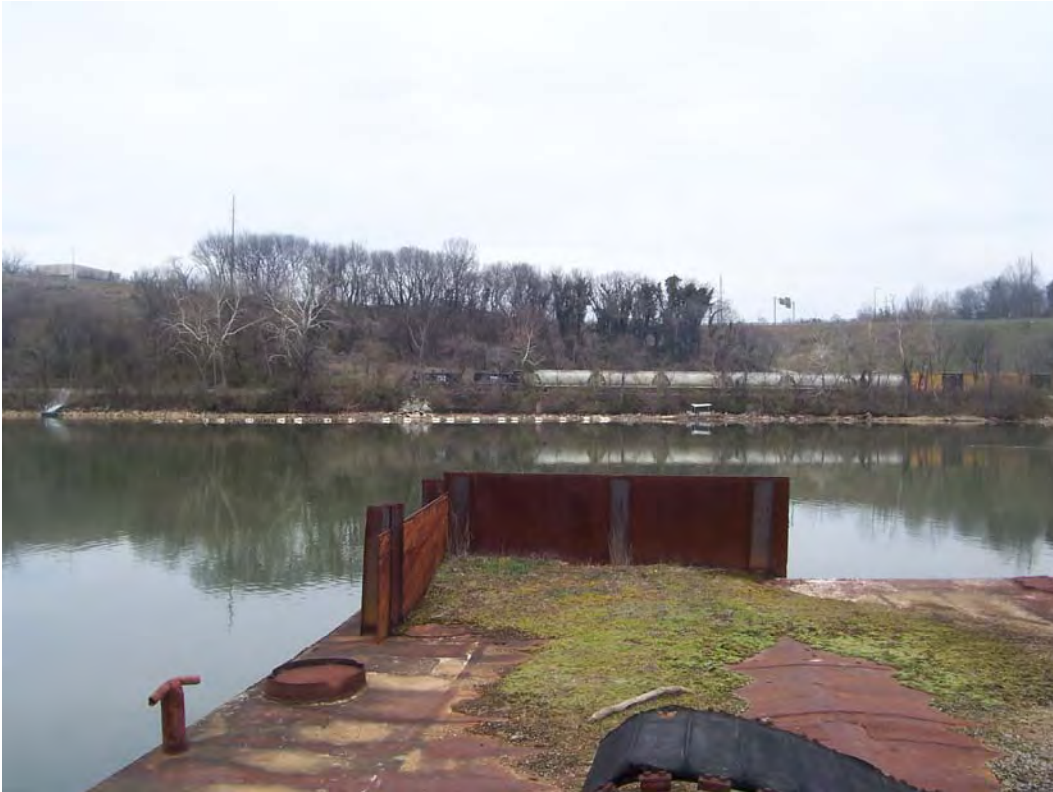
Photograph 10-18. View to north from dock.
