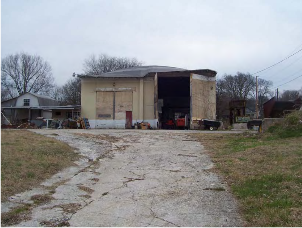
Photograph 10-3. View to south from road to boat ramp.
