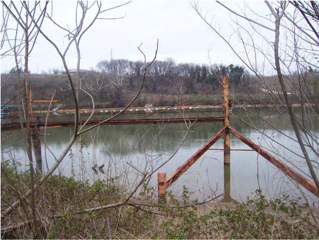
Photograph 10-15. View to north. Metal barge pier.
