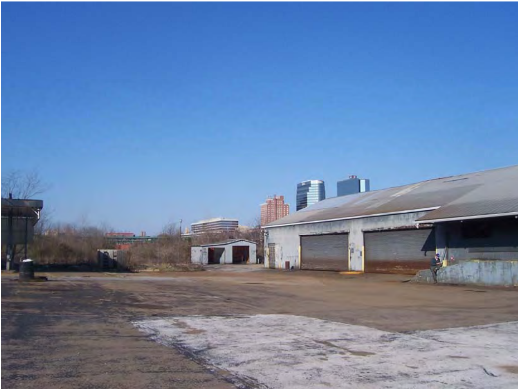
Photograph 9-6. View to northwest. Main building and garage area.
