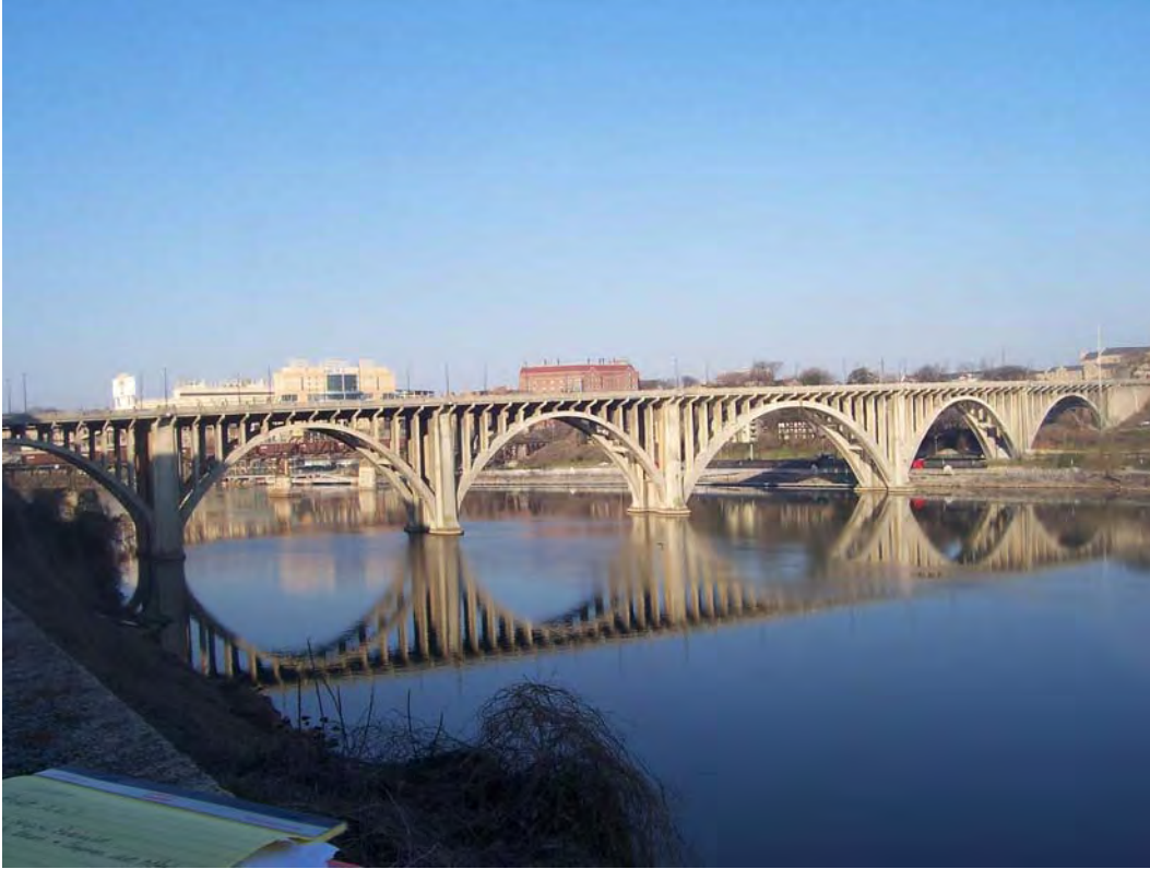
Photograph 6-3. View to northwest from Baptist Hospital of Henley Street Bridge.
