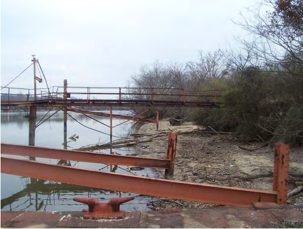
Photograph 10-17. View to southeast from dock of shoreline and metal barge pier.
