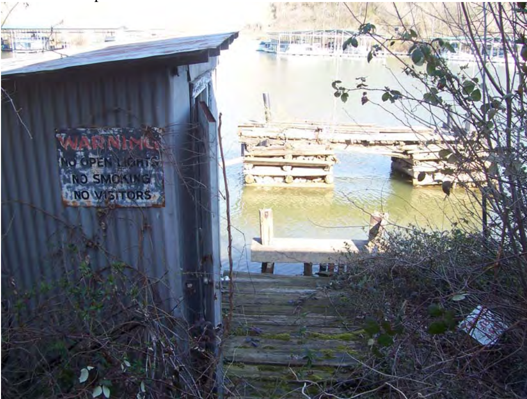
Photograph 9-48. Dock and pump house associated with wooden pier.
