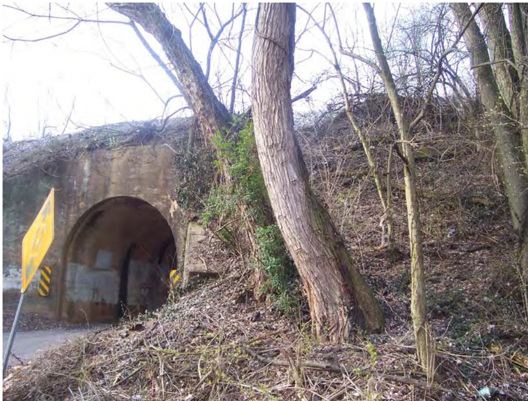
Photograph 1-12. View to southwest. East side of underpass and railroad.
