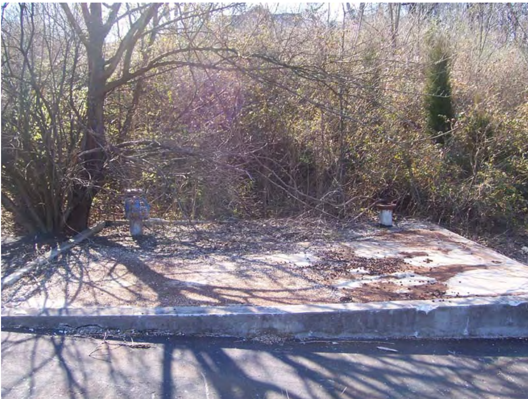
Photograph 9-26. View to south towards Langford Avenue; south of old fueling station.
