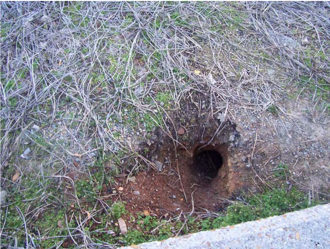
Photograph 6-12. Typical groundhog hole found in bluff area.
