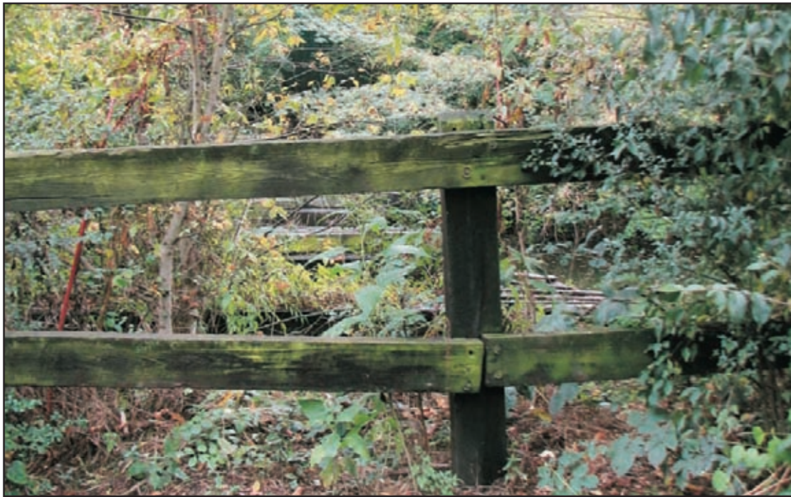
21B. View of Bridge Abutments Crossing Goose Creek
