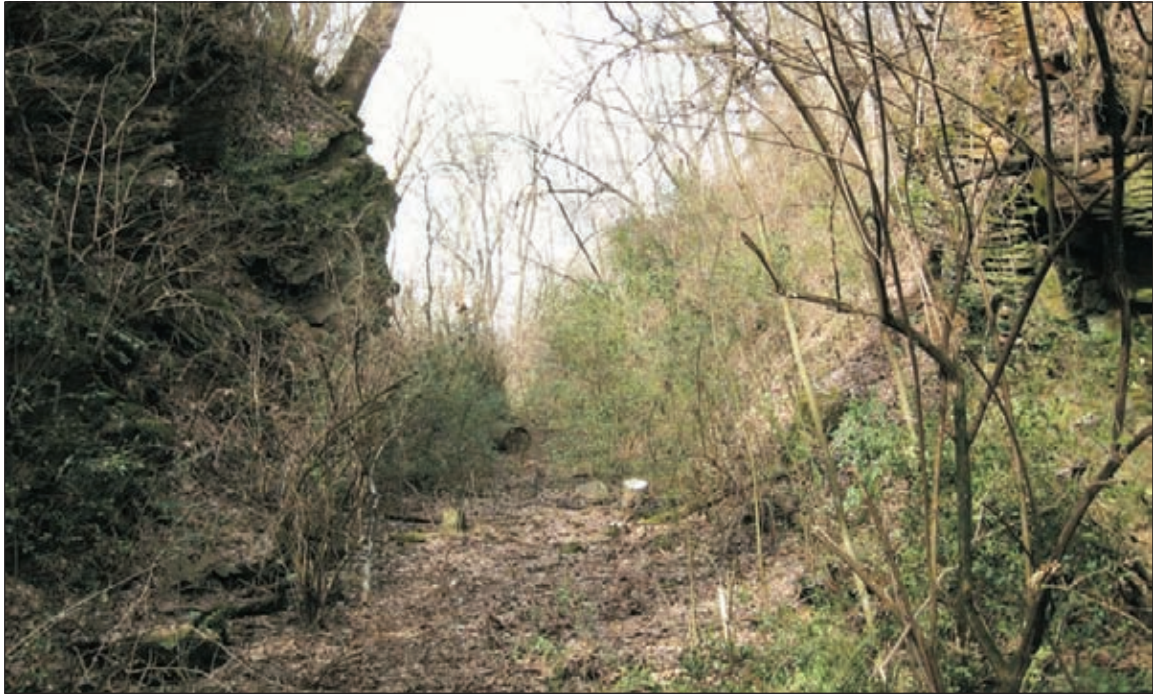
8A. Abandoned Railroad Cutting, Looking North. The Existing CSX Railroad Tracks are on Top of the Cut at Left
