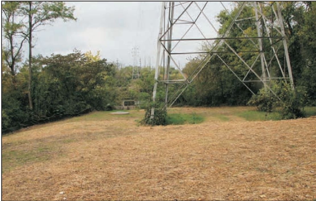
21A. Transmission Lines in Project Area
