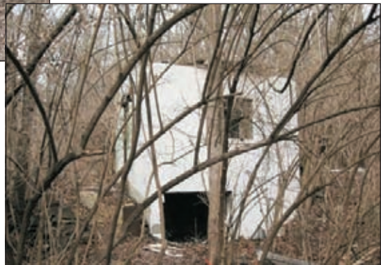
9C. Detail of Cement Block Building, Rear Facade. Looking East
