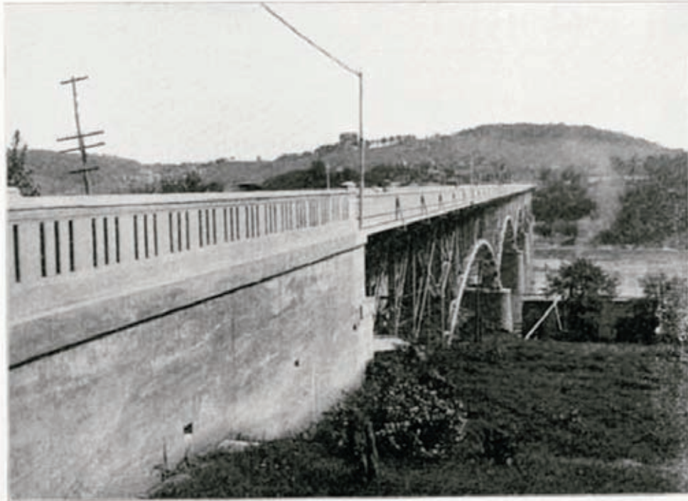
NEW COUNTY BRIDGE ACROSS TENNESSEE RIVER AT KNOXVILLE. Completed July 1st, 1908. 109 feet in length, 42 feet in width, 105 feet above low water mark. cost, all complete, $227,500.
