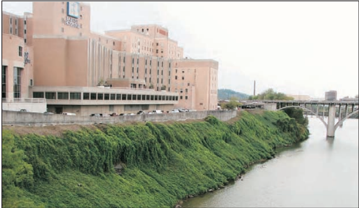
30A. View from the Gay Street Bridge
