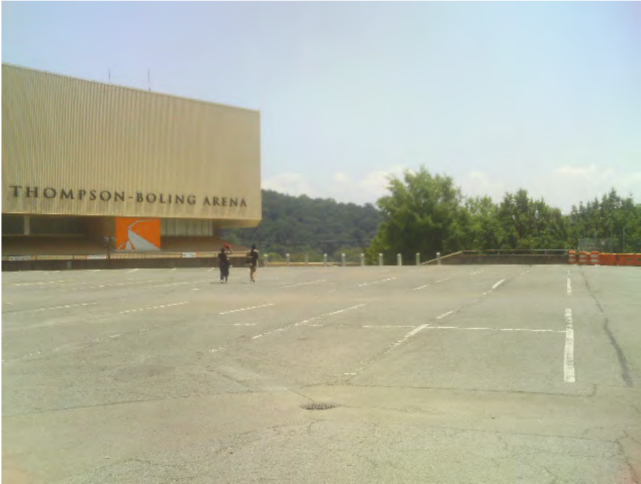
3. Top deck of Thompson Boling Arena facing southeast.
