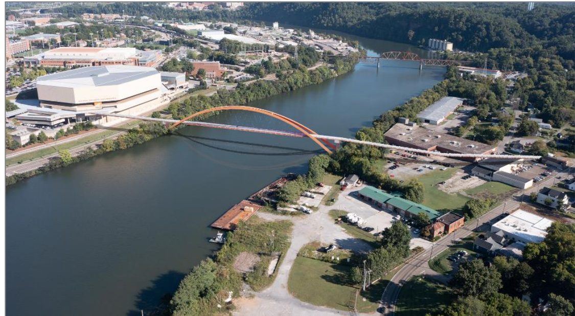
South Knoxville Waterfront Bike and Pedestrian Bridge, bridge rendering prepared by Modjeski & Masters
