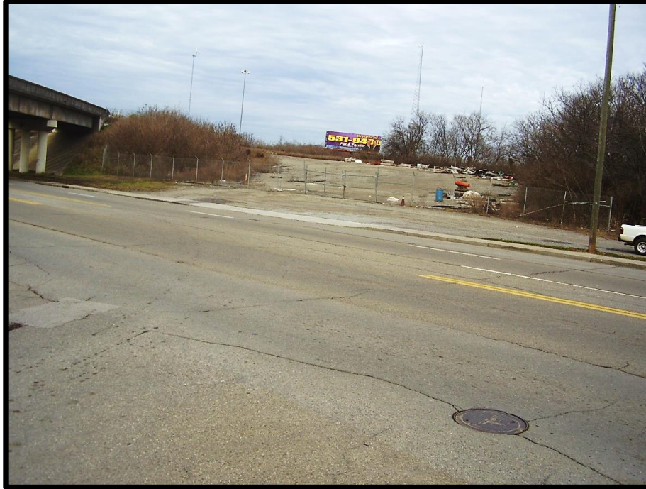
Photograph 1: View to the north of 5th Ave. for potential Blackstock Ave. extension. Area was used for equipment storage during I-275 improvements. Piles of construction material such as barrier walls, trash, and debris still remain.
