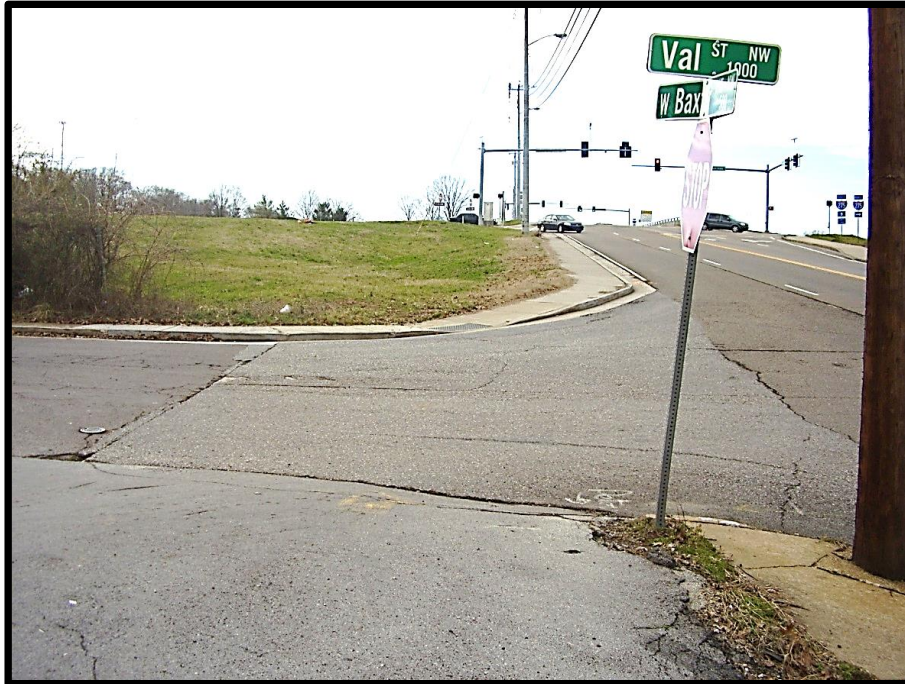
Photograph 13: View to the west of the proposed Marion Street (Val Street) and Baxter Avenue intersection improvements. RSG Roofing Supply Group is adjacent.
