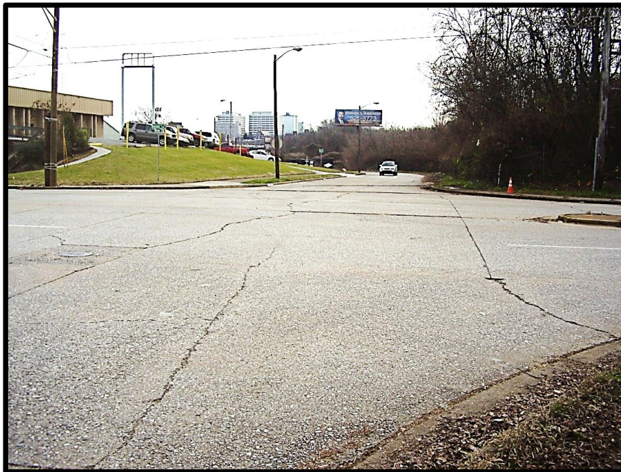
Photograph 10: View to the south of the Blackstock Avenue and Bernard Avenue intersection.
