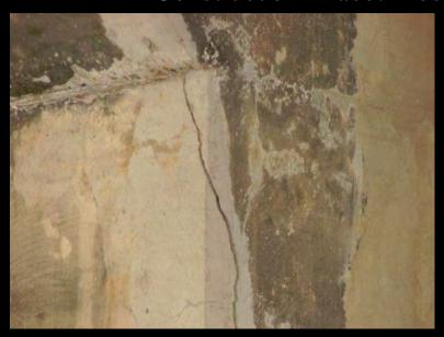
Vertical Cracking Along an Abutment of the Sutherland Avenue Bridge
