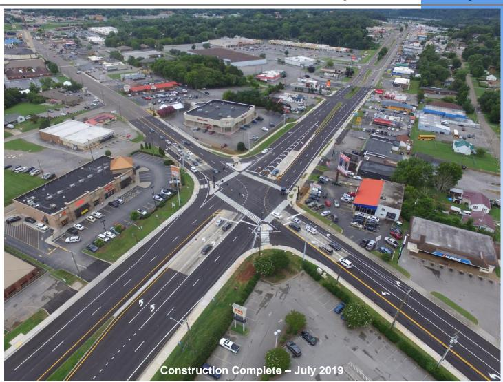
**Project Description:** This project will construct intersection improvements to allow for more efficient turning movements and storage for vehicles, extending sidewalks to provide access to nearby KAT bus stops and adding safer pedestrian crossings with signals and refuge islands. Additionally, gas, water, and sewer lines will be relocated for KUB as part of this project.
