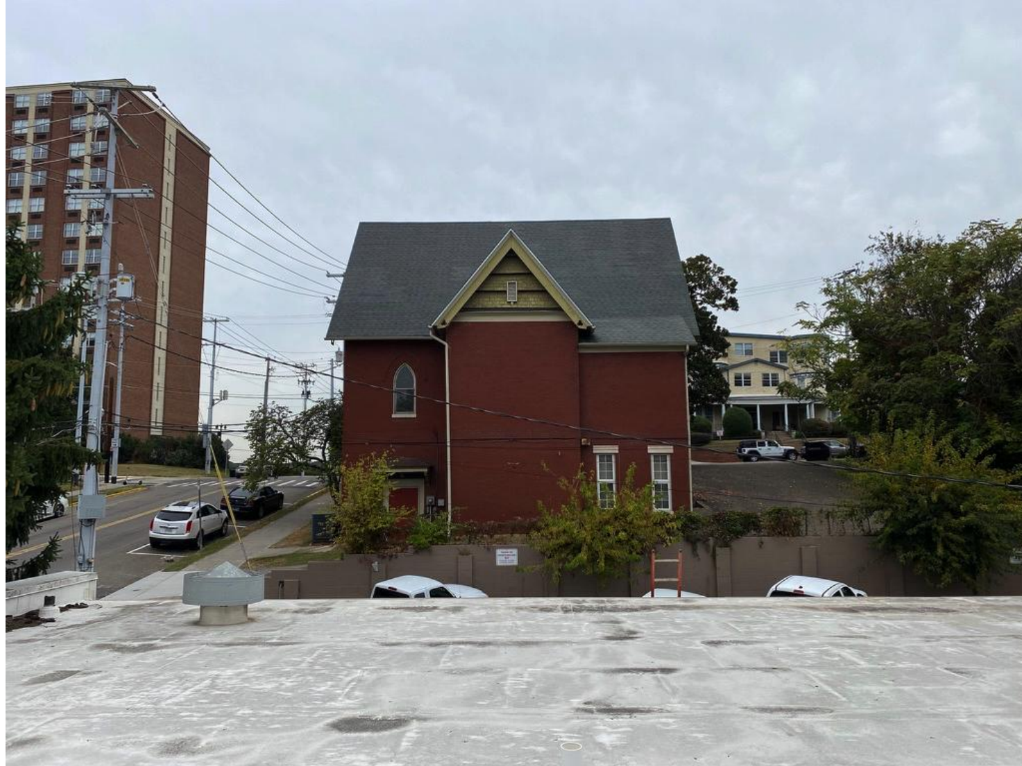
Parking lot and site wall from roof
