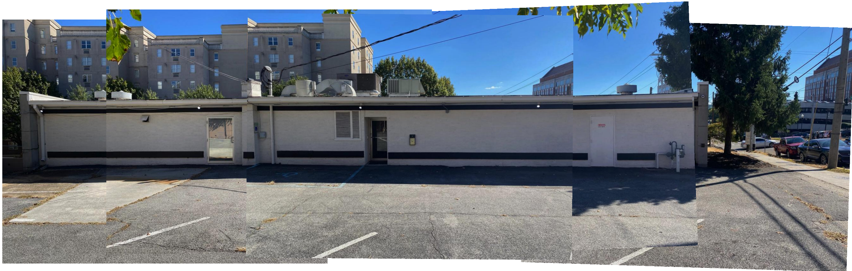
Rear of building from parking lot
