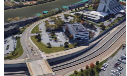
AERIAL LOOKING NORTH
