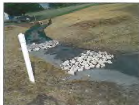
Infiltration trench at Elyria Drive
