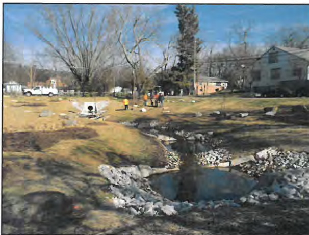
Banks Avenue stream restoration
