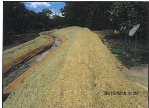
Cavalier Avenue stream restoration
