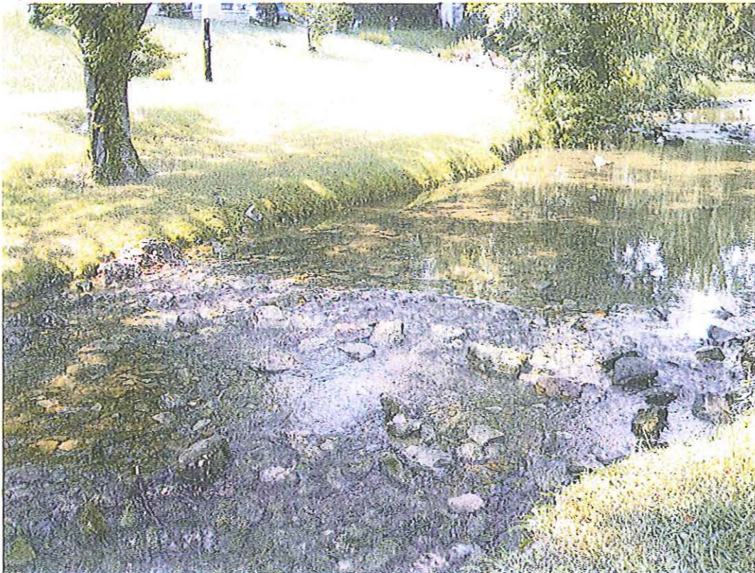
This weir was found and removed by Kirk Forgety on June 13, 2011.
