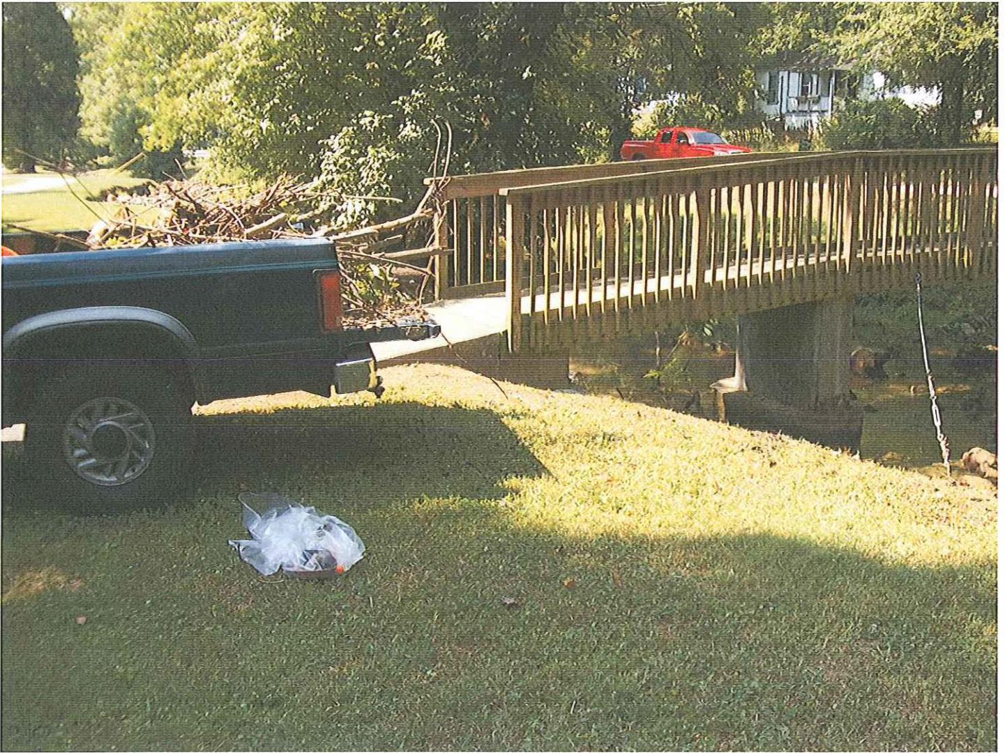
... and then removed from the bank by truck.
