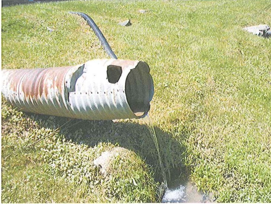
Photo 14. Outfall at First Creek.
