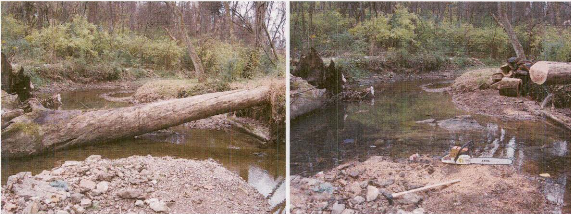
Weir #9 Baker Creek N35 0 57.200' W83 0 53.360'
