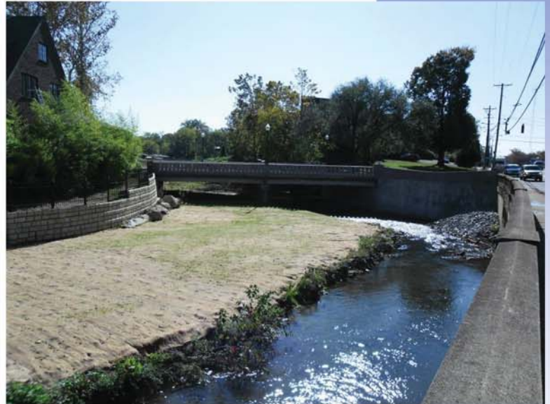
Fairmont Bridge Construction Complete
