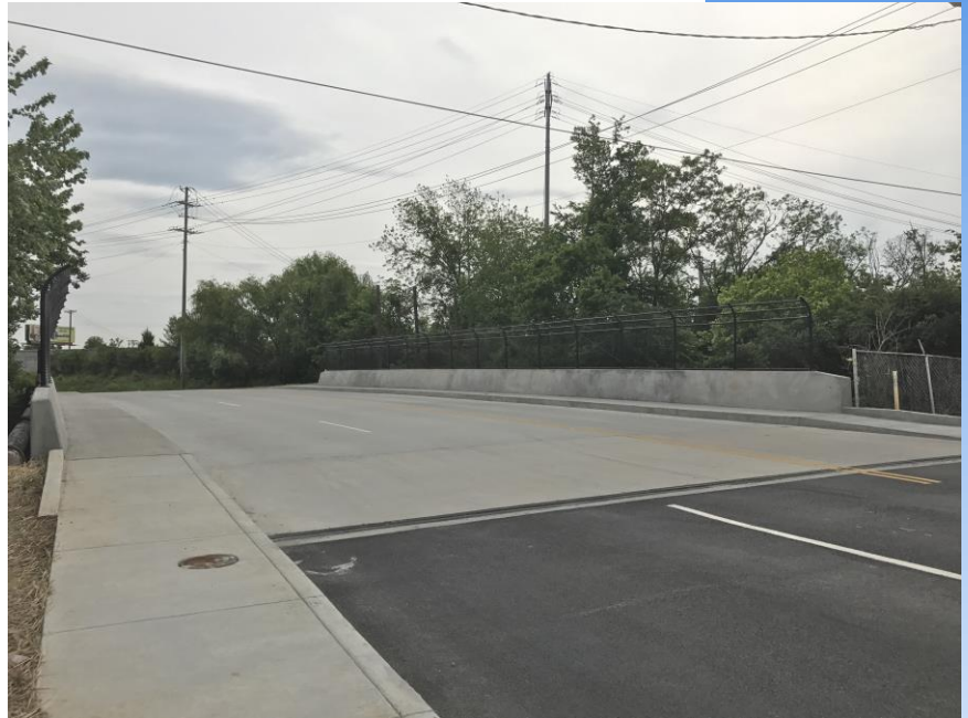
Construction Complete - May 2017
