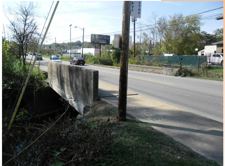
Sutherland Avenue Bridge Looking West
