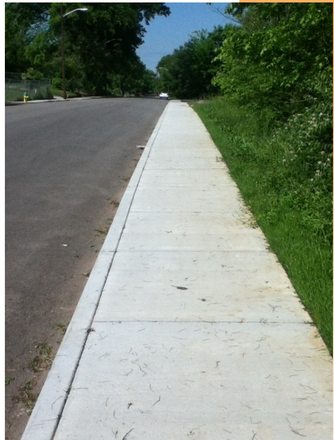
Linden Avenue After Construction
