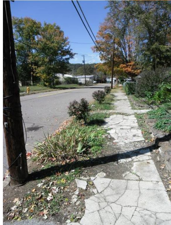
Harvey Street Looking Northwest
