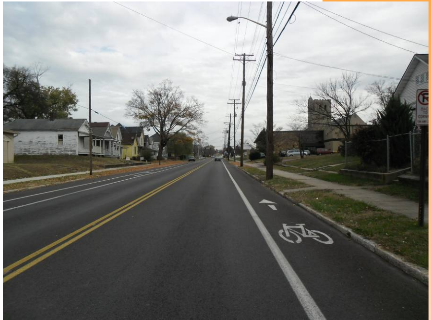
New Pavement Along Baxter Avenue
