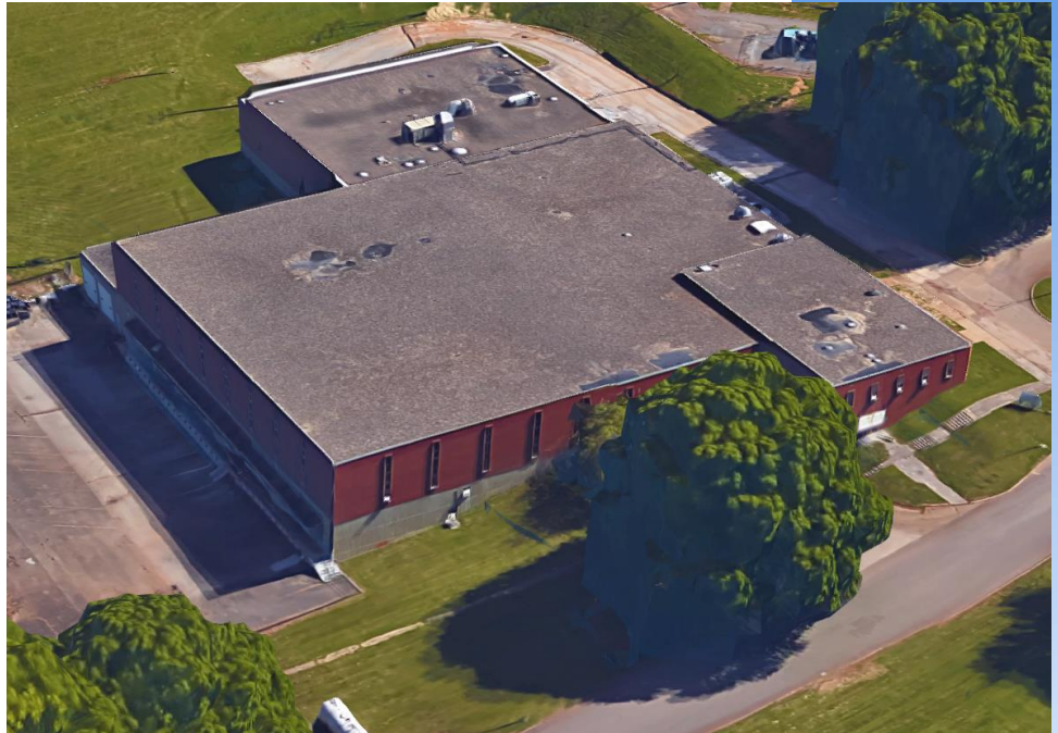
Lakeshore Central Service Building
