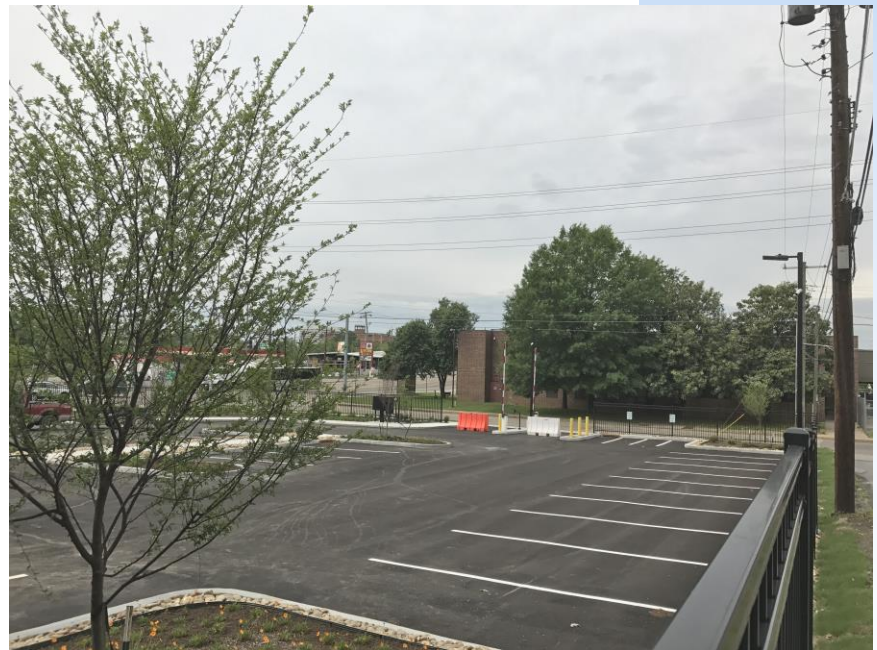
Construction Complete – February 2017
