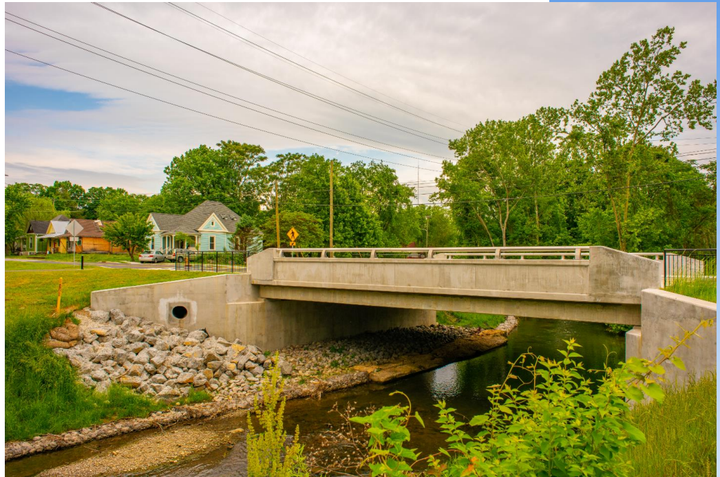
Construction Complete – May 2019
