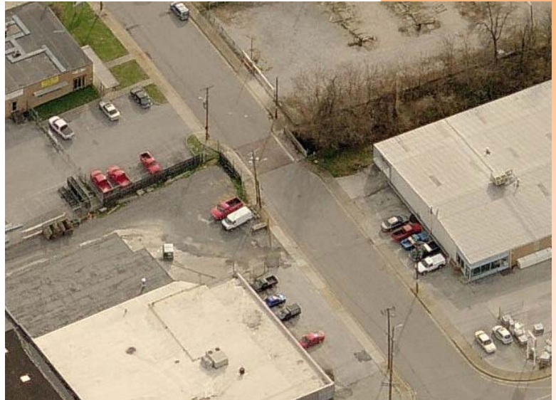
Georgia Street Bridge – Looking South
