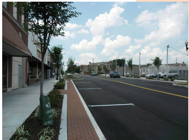
N Gay Street - (Looking North After Construction)
