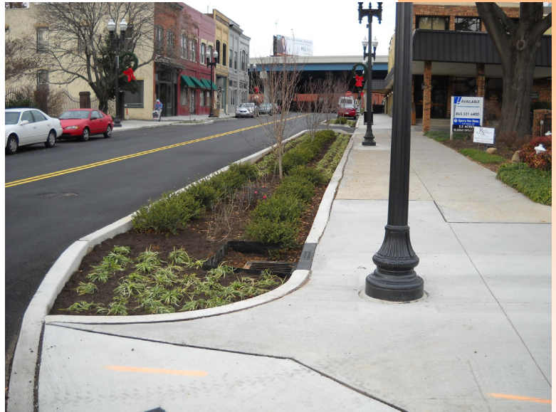
300 Block Looking North – Construction Complete
