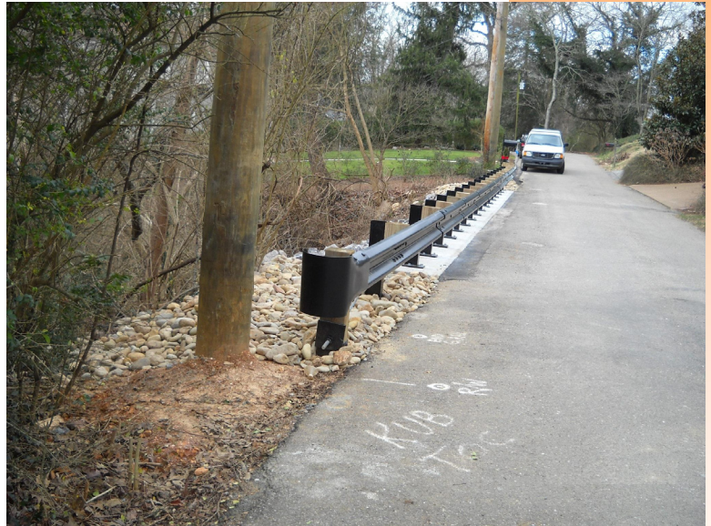
Eutaw Place Looking West –Construction Complete
