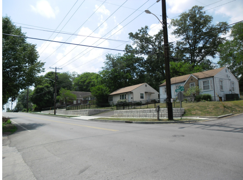
Wall Near Kenyon Street & E. Woodland Avenue Looking West - After Construction
