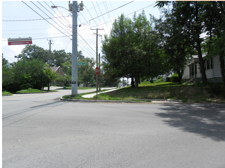
Huron Street at E. Woodland Avenue Looking West - After Construction
