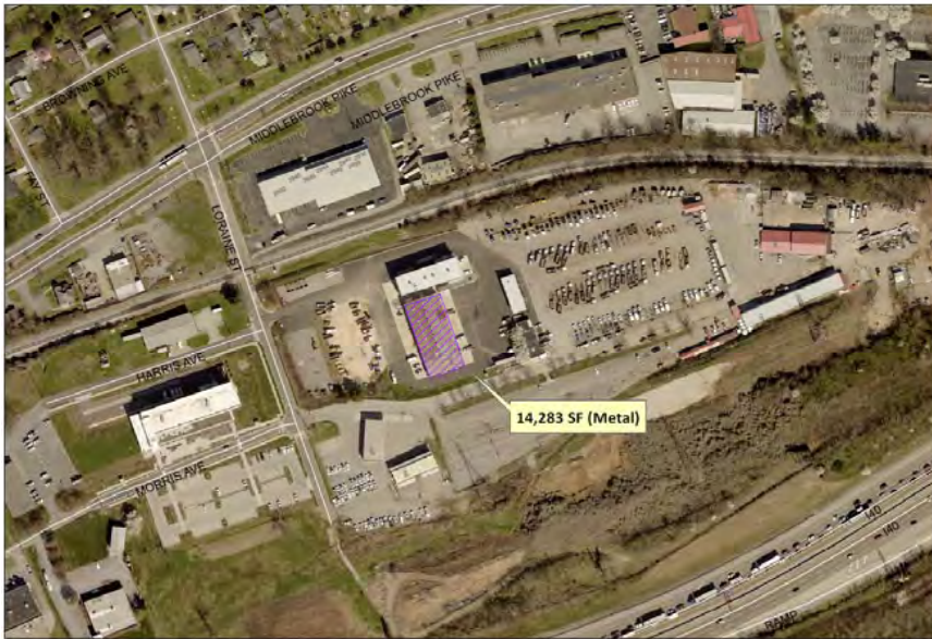
Knoxville - Knox County - KUB Geographic Information System Loraine Street Heavy Shop Roof 1 inch = 200 feet
