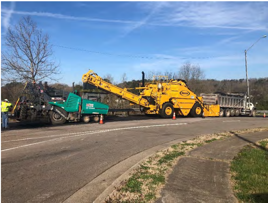
Shuttle Paving Operation Along James White Parkway
