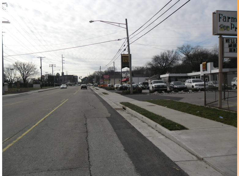
Sutherland Avenue at Pilot Food Mart Looking West – Construction Complete
