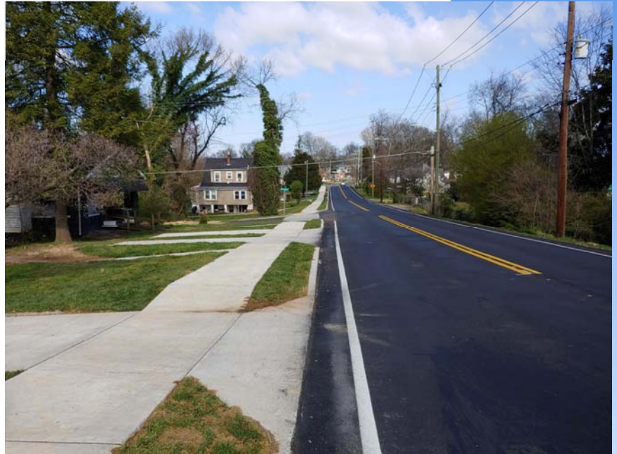
213 S Castle Street Looking North – Construction Complete
