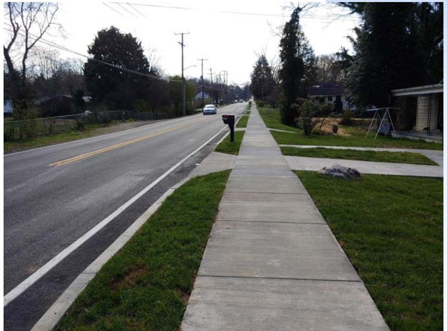
205 S Castle Street Looking South – Construction Complete
