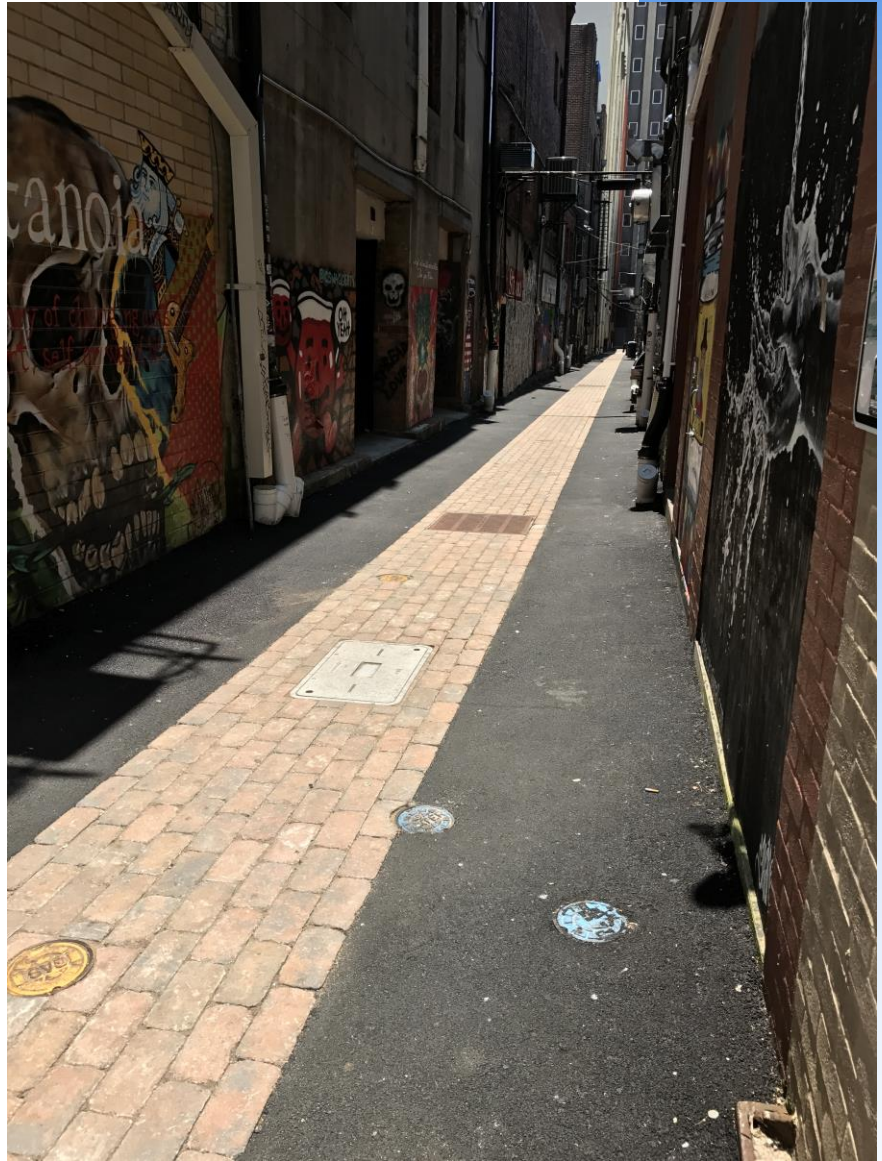
Strong Alley – Looking South Construction Complete – July 2017
