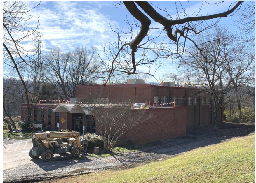
During Construction – December 2020
