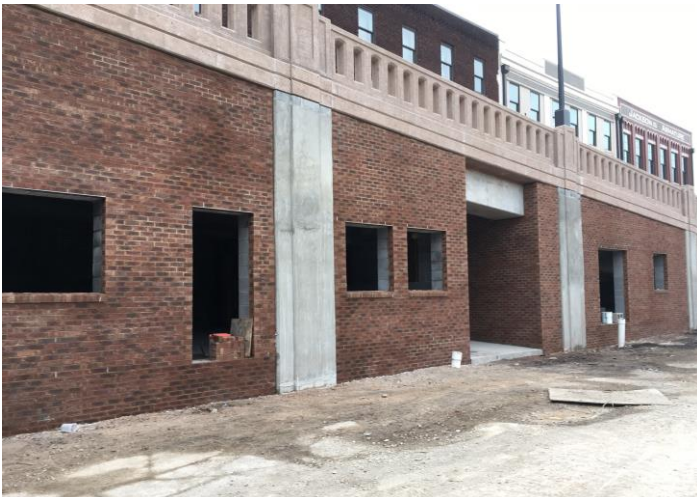
West Ramp – January 2021
