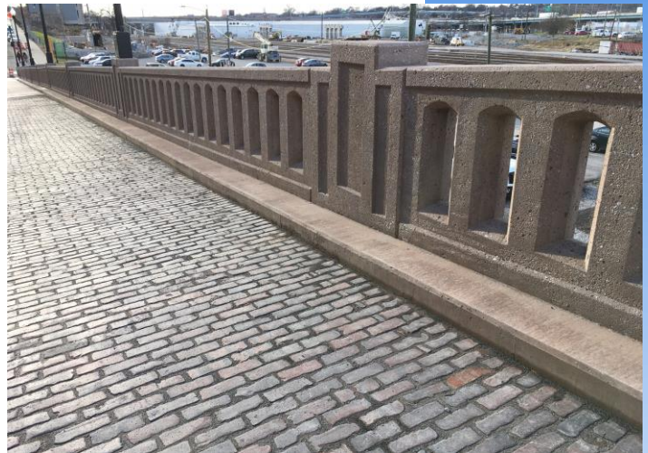
Original Pavers on New Ramp – January 2021
